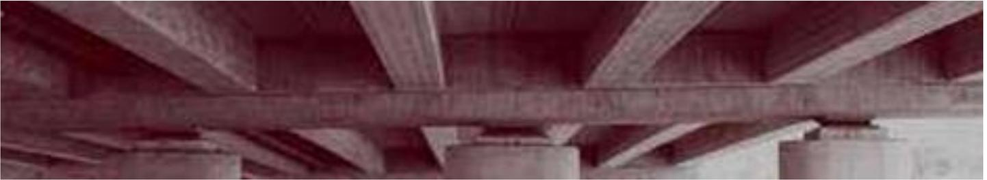
Cast-in-place pan joist slabs can provide economical concrete roof and floor construction. They are cast above reusable metal pans, foam panels, fiberglass or plastic pans, concrete or clay tiles, or other forms. The reusable pans are most frequently used. The ribs may run in one or two directions. This slab construction is generally known as "one-way pan joists" or "two-way pan joists".
