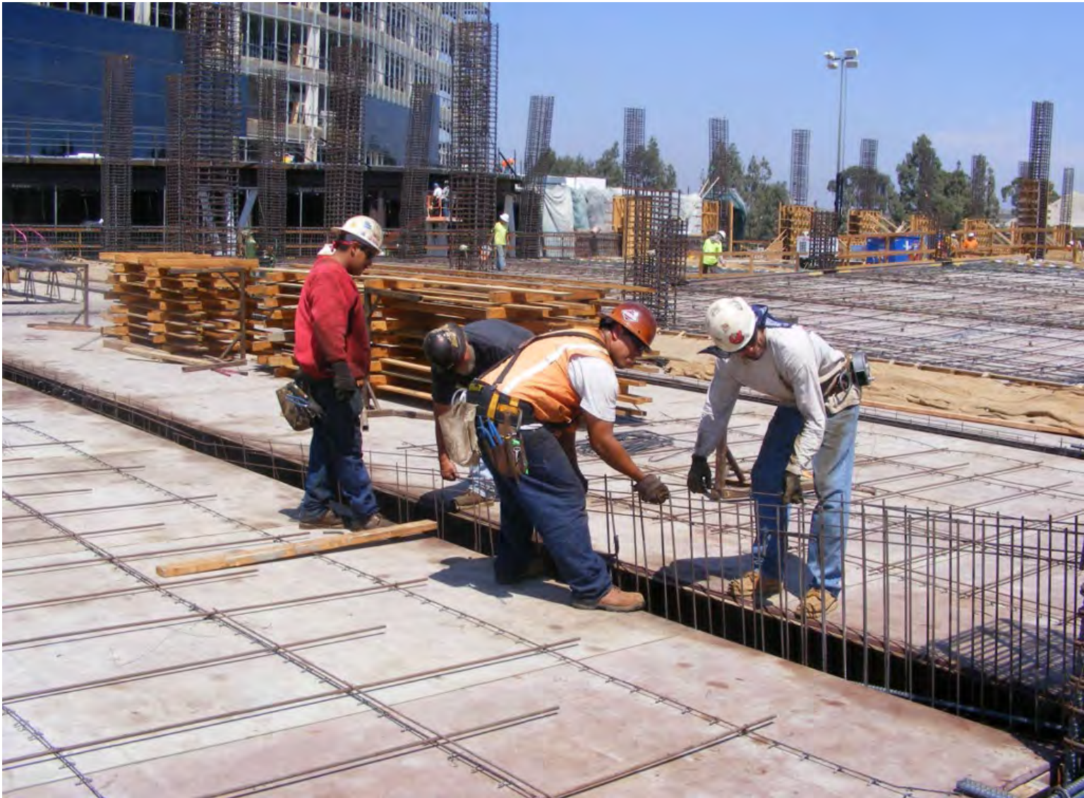
Placing crew setting beam stirrup cages in post-tensioned beam. Notice the slab reinforcement mats already in position, comprised of prefabricated WWR mats containing staggered wires per the design professional's detailed requirements.
