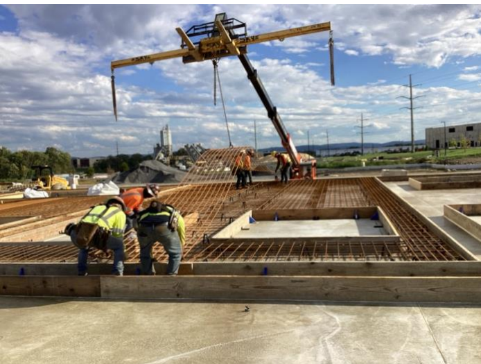
Figure 6: Telehandler forklift and spreader beam
