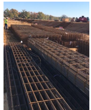
Figure 7: WWR material bundles in lay-down area
