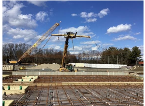
Figure 5: Telehandler forklift and spreader beam
