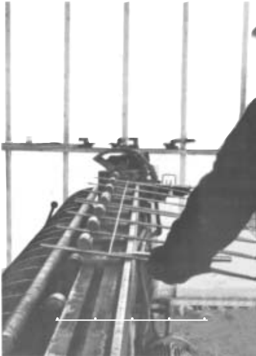
START: Workers feed sheet of welded wire under mandrels.
