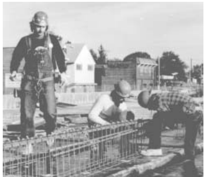
Placing Stirrup
