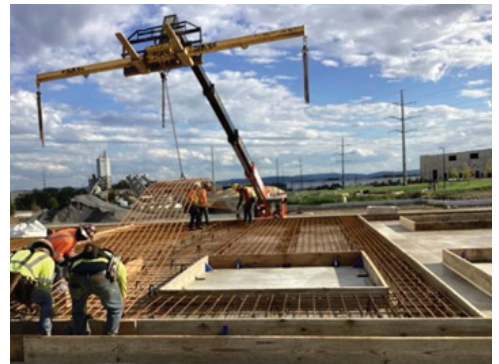
Figure 6: Telehandler forklift and spreader beam
