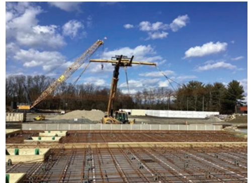
Figure 5: Telehandler forklift and spreader beam
