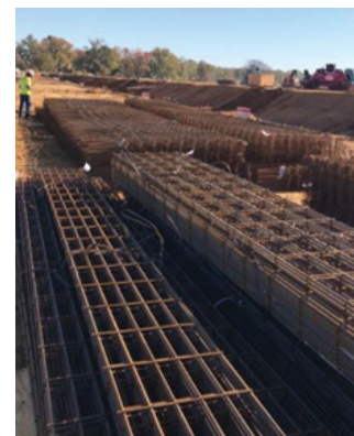
Figure 7: WWR material bundles in lay-down area
