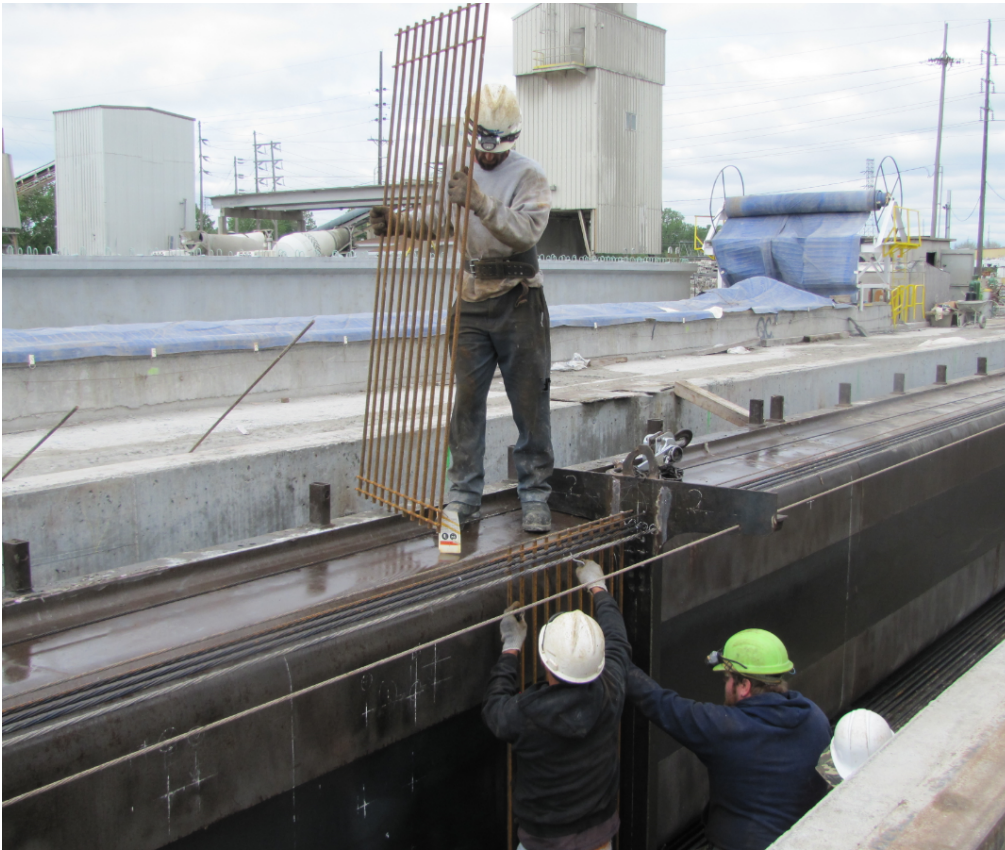
Figure 57: A placing crew installs WWR stem reinforcement in a casting bed for a precast prestressed highway bridge girder.
