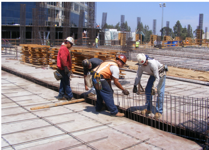
Figure 2: A placement crew installing a bent WWR mat for use as shear reinforcement in a post-tensioned concrete parking garage beam. Also note the flat WWR mats already placed for use as minimum mild steel reinforcement in the structural slab that will span perpendicular to the beams.
