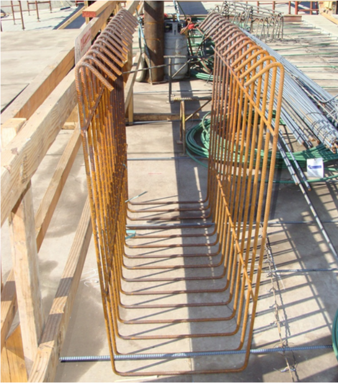
Figure 40: A bent WWR mat with 135-degree hooked terminations for use in the beams of special moment frames (high seismic application).
