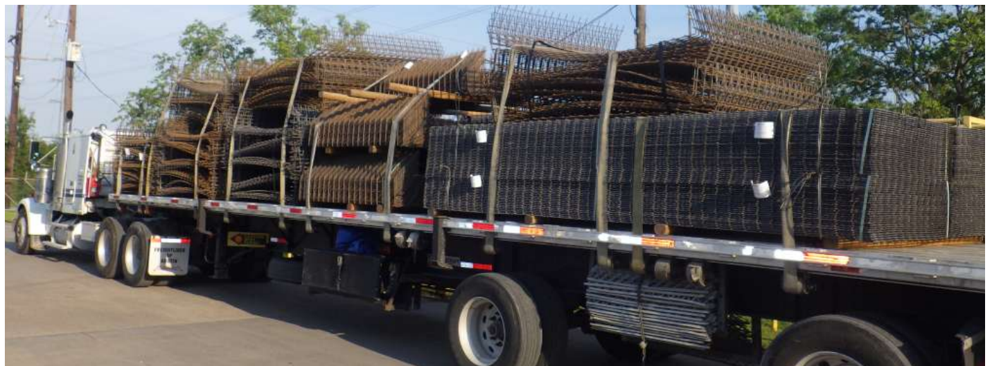
Figure 51: A combination of flat and bent WWR loaded on a truck, ready for transport. Placement of the various WWR mat bundles is carefully planned to maximize the amount of material that can fit on the truck without incurring violations related to dimensional and/or weight restriction.
