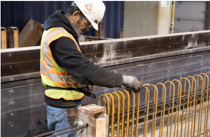
Figure 55: A worker checks the positioning of bent WWR mats in a casting bed for a precast prestressed girder.
