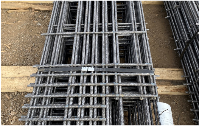
Figure 11: WWR mat bundle showing variable spacing of linewires and crosswires
