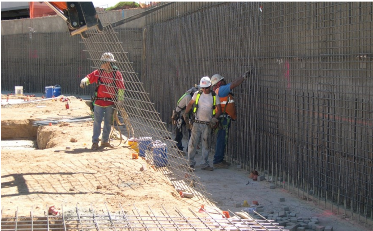
Figure 56: Workers utilize a telehandler to assist in the placement of WWR wall mats.
