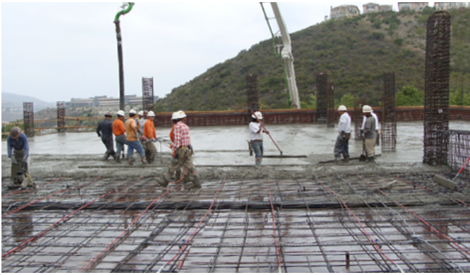
Figure 53: Placement of concrete in a post-tensioned parking deck structure where WWR was used as the mild reinforcement in beams and one-way slabs.
