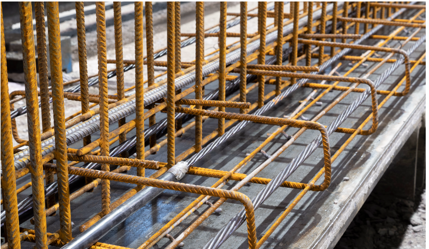
Figure 1.2: Bent WWR in a casting bed for a precast prestressed highway bridge girder
