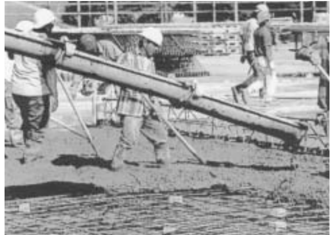
WWR sheets retain their flatness and do not deflect when placed on appropriately spaced supports, even during concrete placement.
