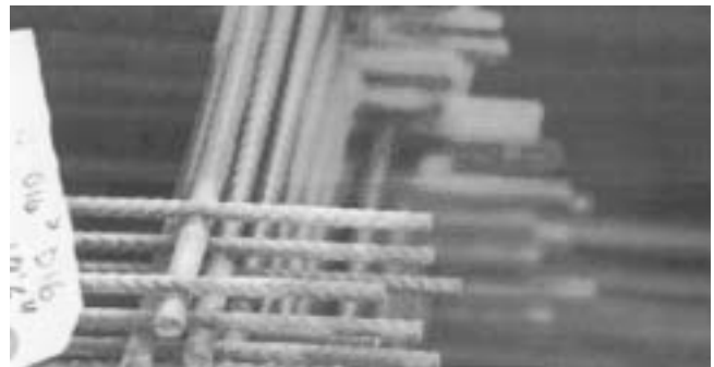
Note that two smaller close-wedge wires provide greater splice efficiency.
