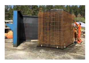
When WWR is used for wall reinforcing, form support accessories are available to hold the sheets of WWR in place to provide the necessary cover.
