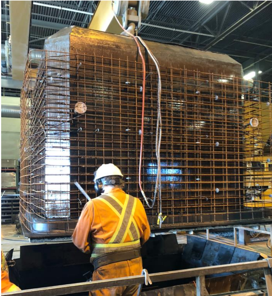
An assembly of WWR mats around the inner core form.
