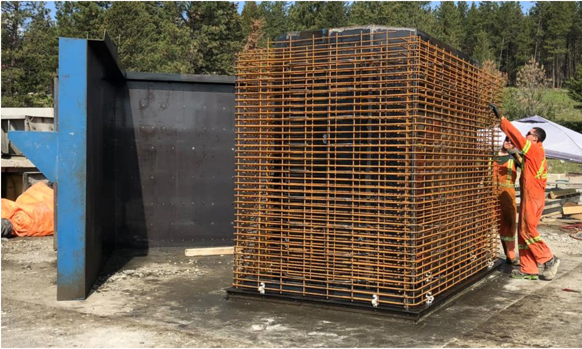
An assembly of WWR mats around the inner core form with a portion of the outer form visible
