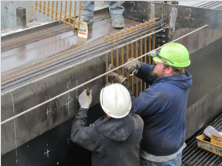
A close-up view of placement of WWR stem mats
