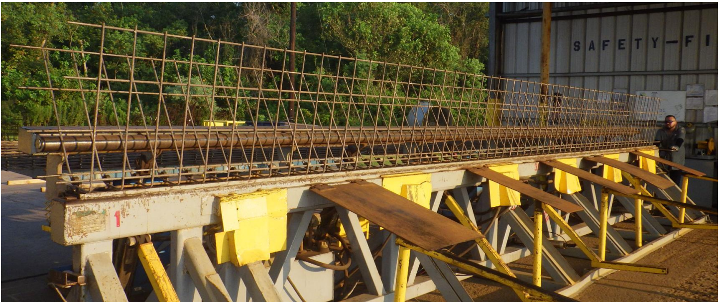
A WWR mat to be used in a roadway barrier is bent on a hydraulic bending machine.
