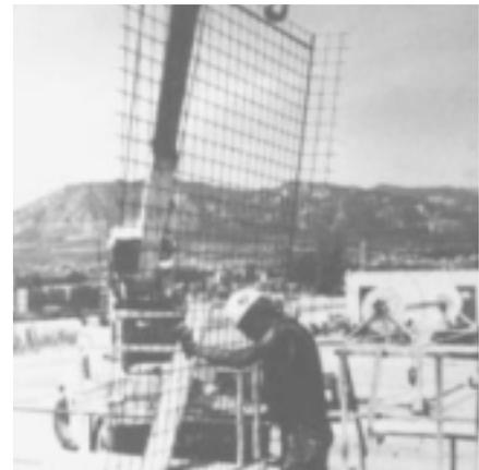
WWR allows the designer to vary the spacing, frequency and pattern of wires to meet exact cross-sectional steel areas for specific applications. Specifying high strength WWR will save up to 25% of the weight of conventional reinforcing, therefore providing significant cost savings on the final project.
