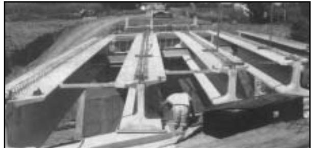
A bridge on Highway 8 in Salem, Neb., uses girders that were designed and fabricated in metric. A second metric girder bridge is in the works.
