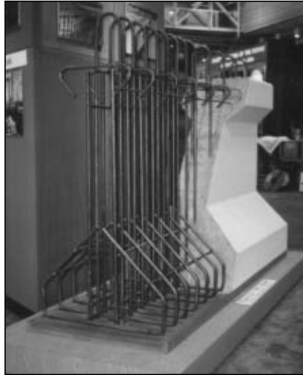
There are many precast and cast-in-place concrete components for bridges and highways. Welded wire can be epoxy-coated to meet the various DOT's requirements in coastal or snowbelt states.
