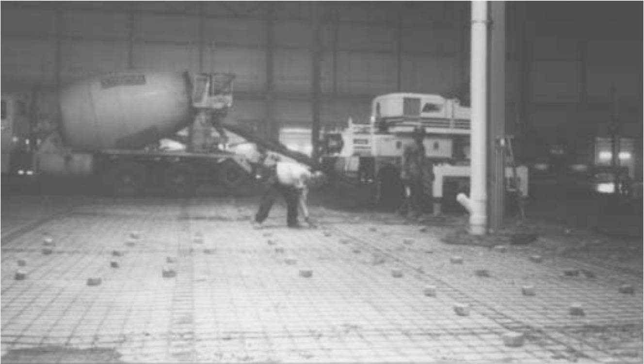
The result is a slab on grade with an exceptional surface quality with minimal intermediate cracks. Shrinkage at the majority of the floor panels occurred at saw-cuts. Minimal curling and no detectable displacement were due to the presence of welded wire reinforcement and overseeing that it was properly positioned. The reality is a properly reinforced, quality slab-on-grade that will save the owner future maintenance and possible costs accrued for shut-down if repairs were needed.
