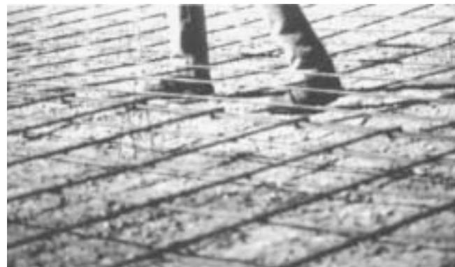
**REMEMBER:** More cost effectiveness and easier placing of WWR can be achieved by using step through styles (12x12 and larger).
