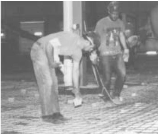
The concrete design specified a 4,000 psi minimum compressive strength mix. The main ingredients were: 6 1/2 sacks of cement, 2% accelerator, and 0.45 w/c ratio with a 4 1/2" maximum slump desired. On-site concrete testing assured that the specifications were followed. Early 3-day compressive strength breaks were over 4,000 psi and many 28-day breaks were over 6,000 psi.
