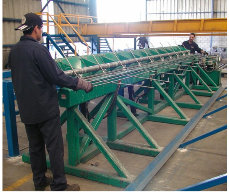
Figure 3-5: Hydraulic or pneumatic machines are used to fabricate WWR bent mats
